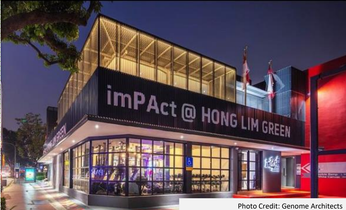
Photo Credit: Genome Architects
